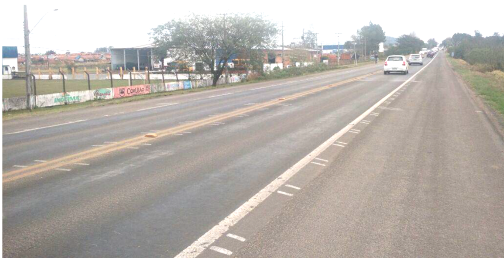
Figure 1. Retroreflectivity reading points for retroreflectorometer positioning
